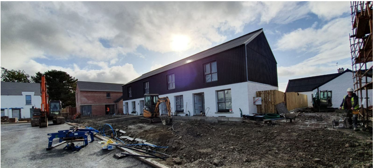
Rural Housing's energy efficient social homes at Lismore Park, Sion Mills are the first to incorporate elements of Rural's groundbreaking new Design Guide for Rural Homes.
